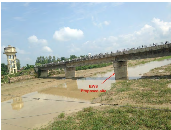
Fig. 9: Flat River with concrete bridge where EWS can be established in the pier of bridge.
